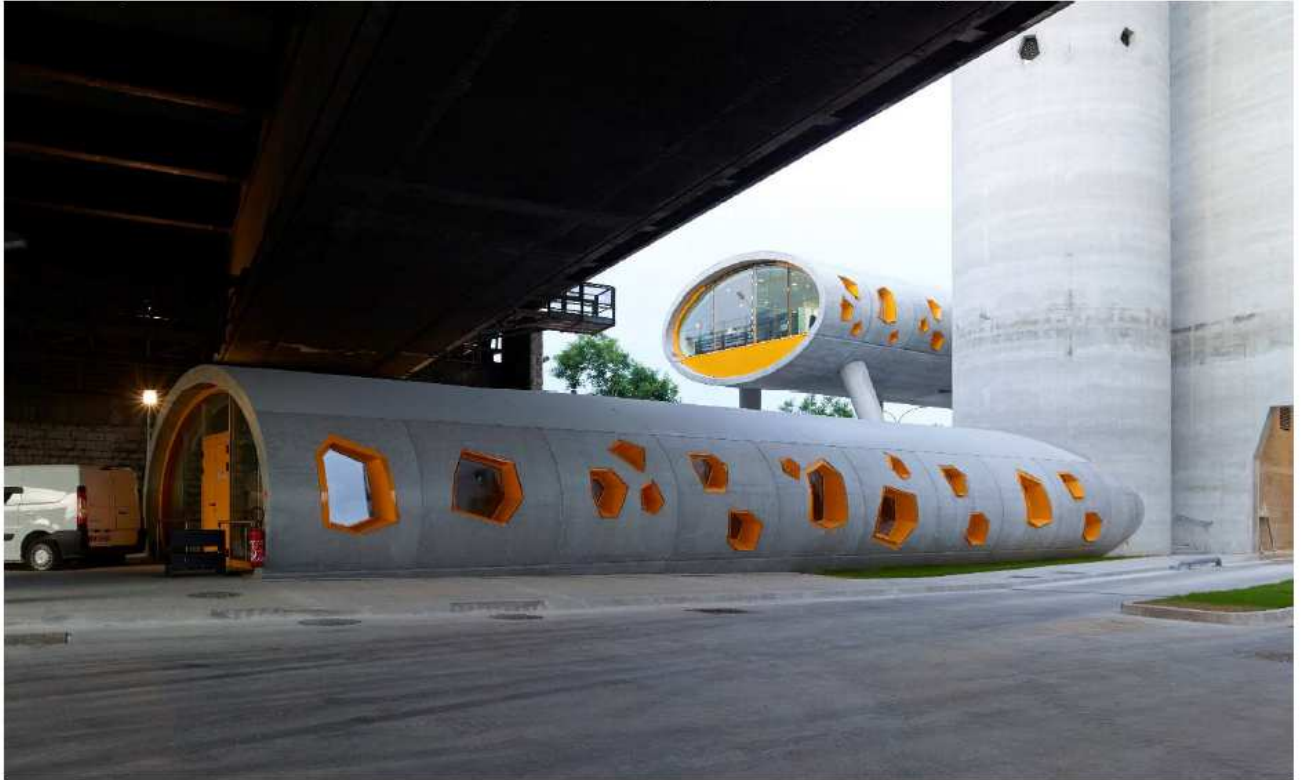
Photo 3: [Under the ring road - VIB architecture - ©Stephane CHALMEAU]
