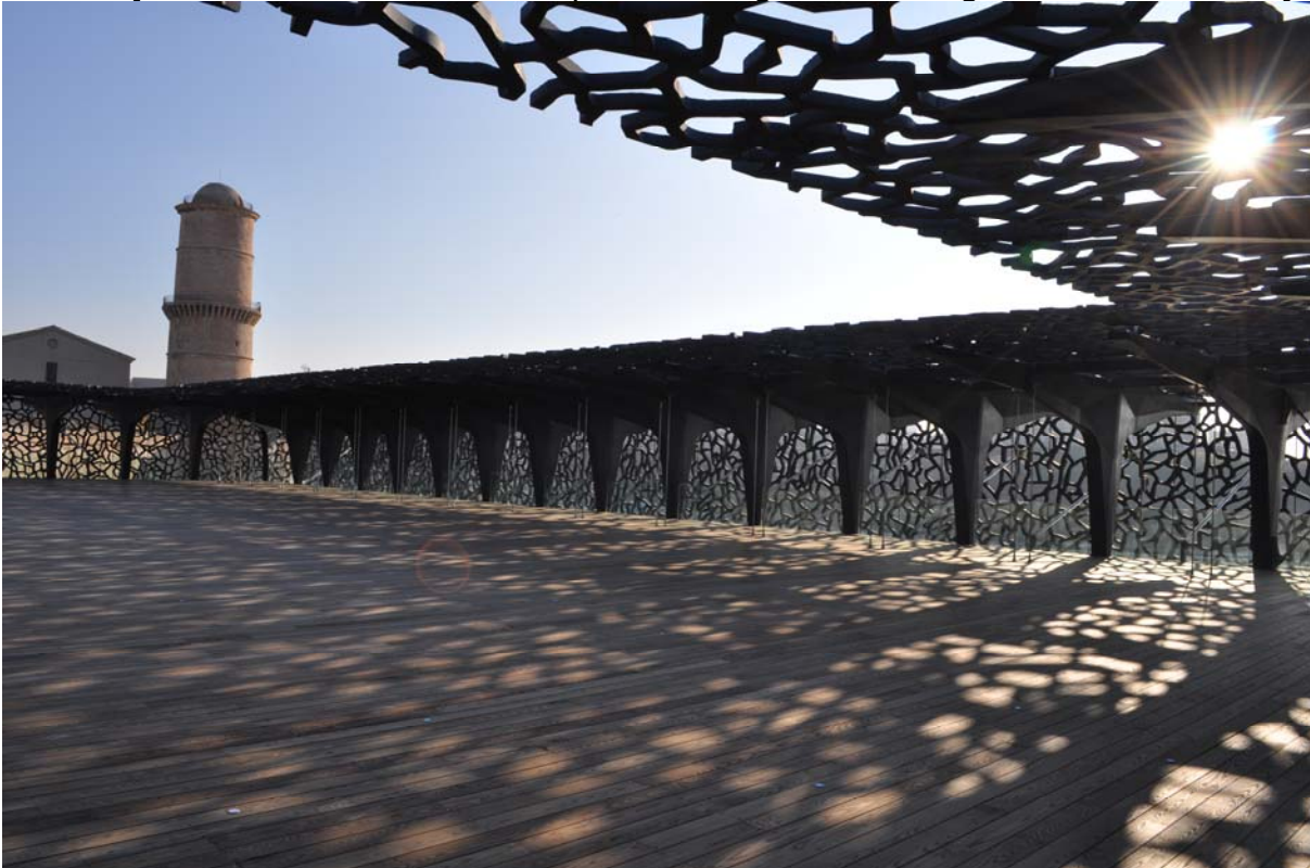
Photo 7:[ UHPFRC brackets and net panel roofing and cladding around the terrace ]
