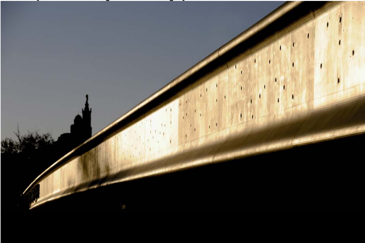
Photo 3:[ UHPFRC facings: the footbridge ]
