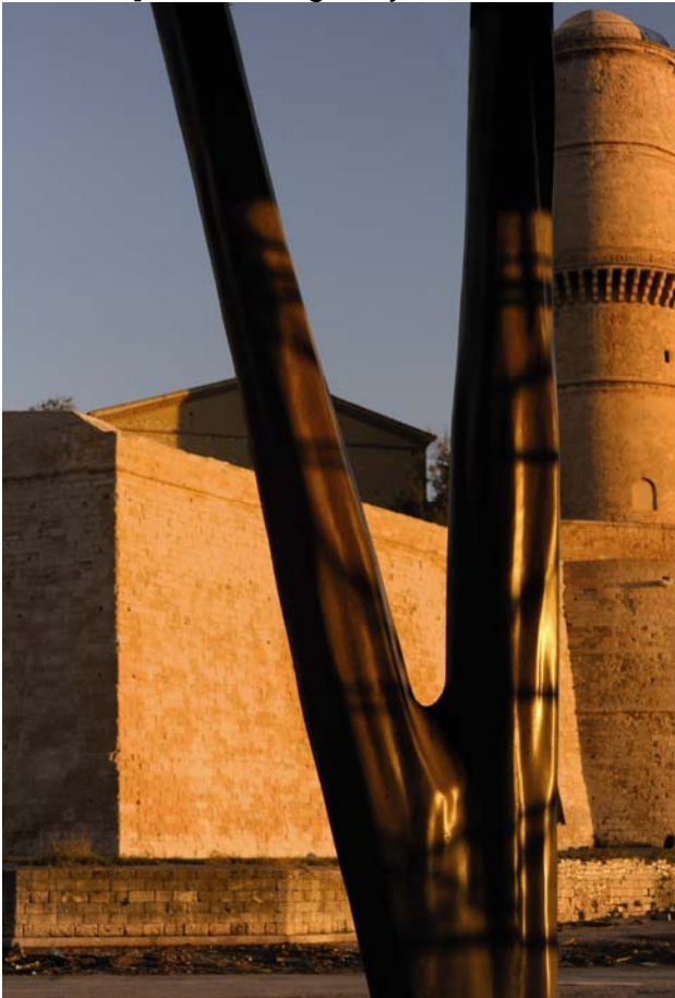
Photo 4:[ UHPFRC glossy formed surface of the tree-shaped columns ]
